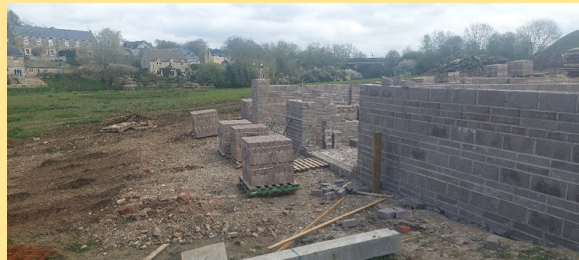
Entrances and internal walls. Photo: Campbell Ritchie
