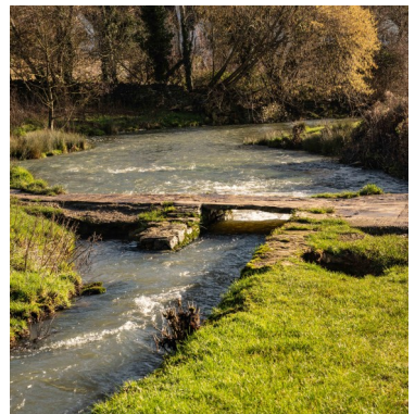
Clapper Bridge near Daniel's Well
