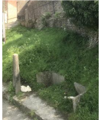
Broken bench slab above the Maltings
